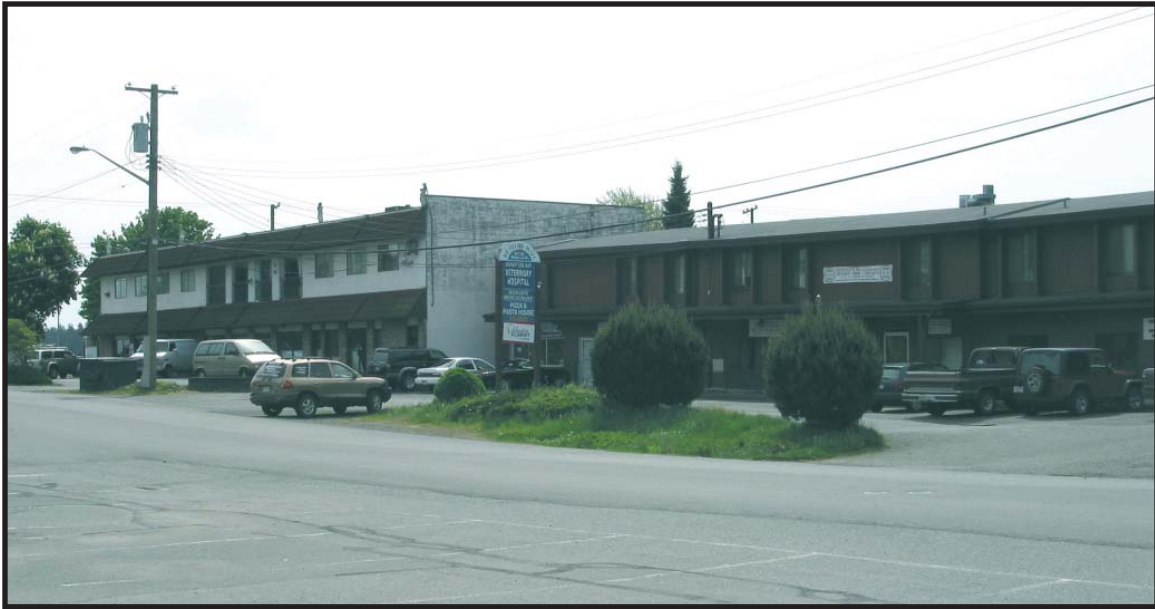
Commercial Development on Wingrove Street
